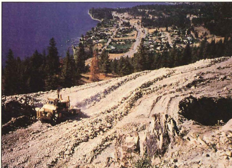
Placing rockfill
